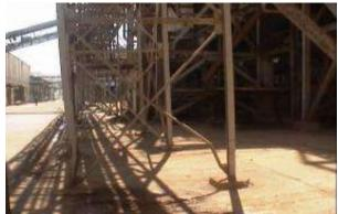
Figure 7 Deformation of bracing system and buckling column.
