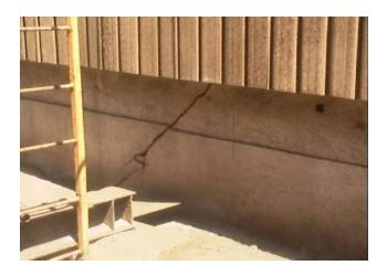
Figure 9 Cracking 45 degrees to both directions and both side of joint.
