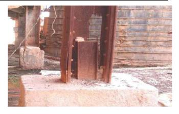
Figure 3 Corrosion of columns.
