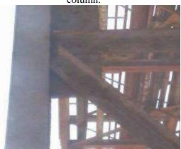
Figure 8 Lack of bolts in the assembly system.
