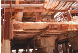
Figure 5 Damage in beams and floors.
