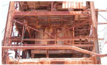
Figure 2 Damage in the bracing system.
